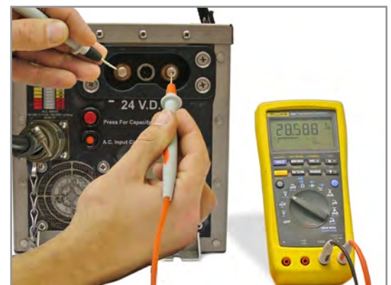
Figure 7.2.3 – Testing DC Receptacle
